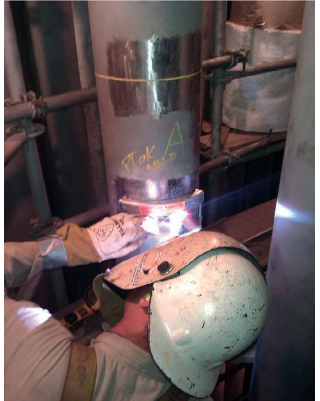
Trained specialist installing sensor
