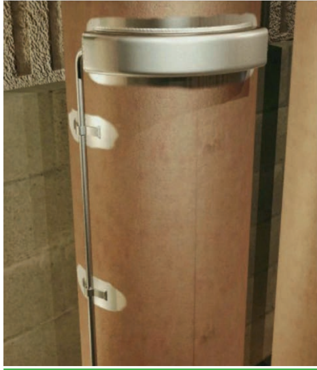
Proper routing with clips
